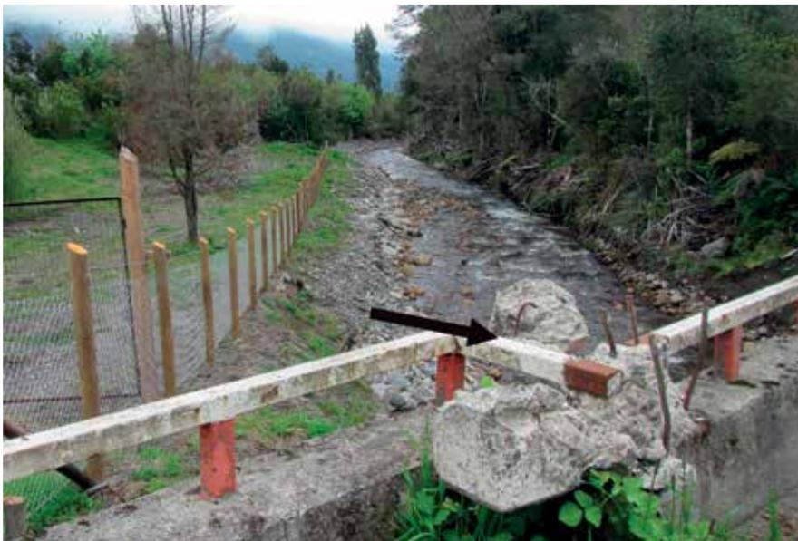
▲ Figure 8. Impact and damage in the Correntoso bridge by 2015 Calbuco lahars.
