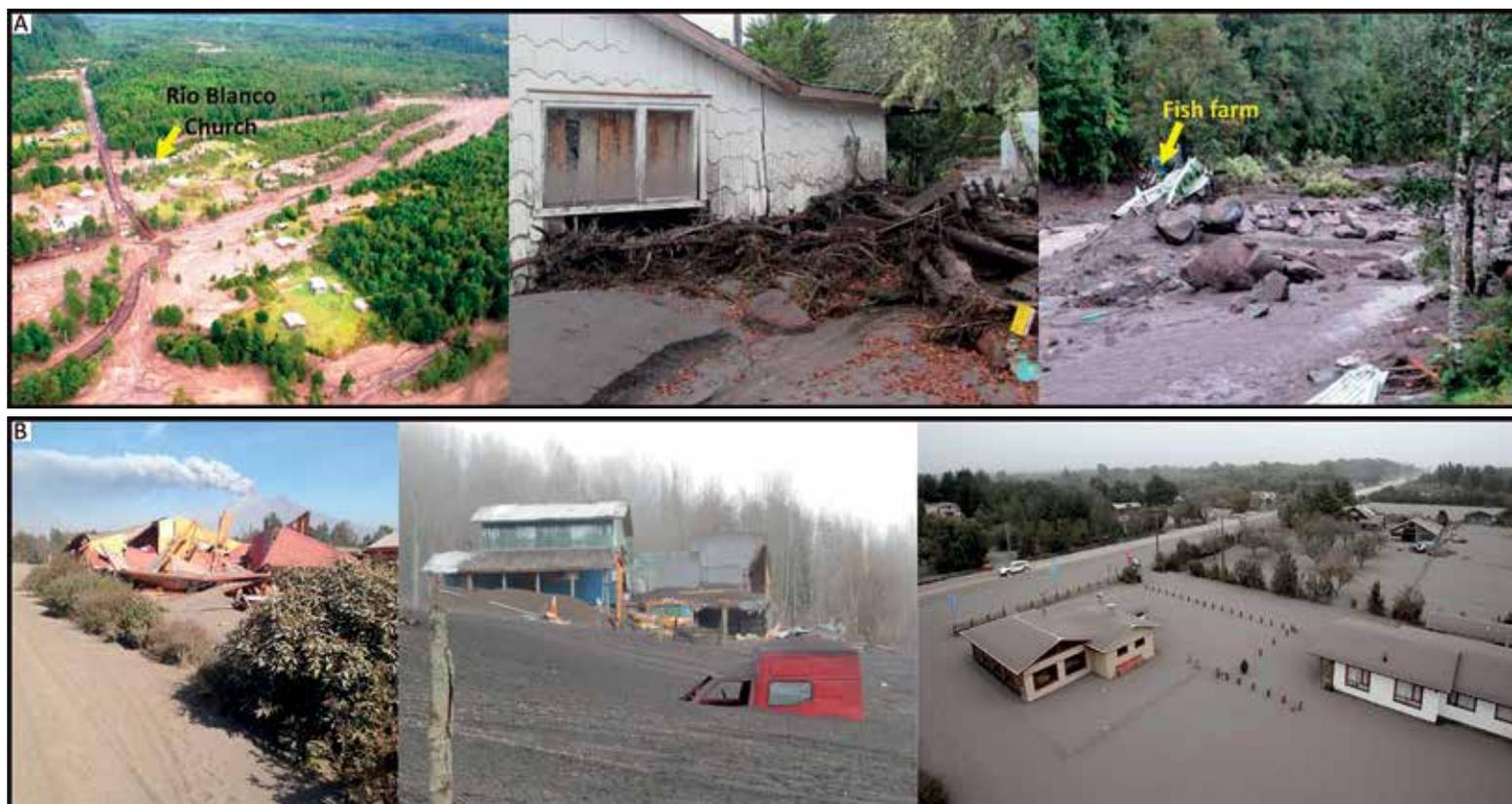
◀ Figure 4. Impacts of volcanic processes of Calbuco volcano 2015 cycle. **A:** houses, road, bridge and fish farming destroyed by lahars of the Blanco Sur and Pescado rivers, the arrow indicates the position of the Church of Río Blanco and fish farm of Pescado river. **B:** fall of pyroclastic rocks in the town of Ensenada where some houses collapsed.
